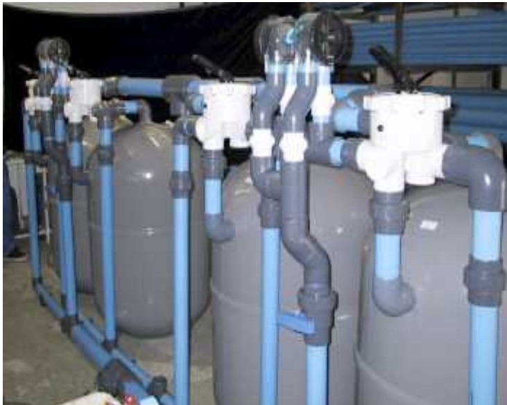
Bank of 4 IF30 Filters with Astral 2" Multi-port valves
